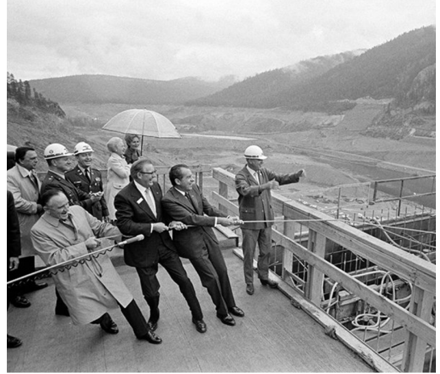
President Nixon at the Libby Dam construction site with Congressman Richard Shoup, Senator Mike Mansfield, and Stanley Stearns, the Libby Dam Project Manager. Photo courtesy of the Richard Nixon Library via Twitter.
