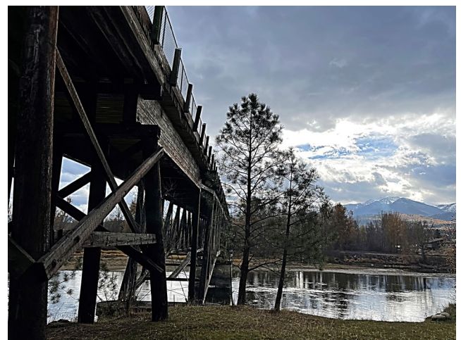
Walking bridge over the Kootenai River
