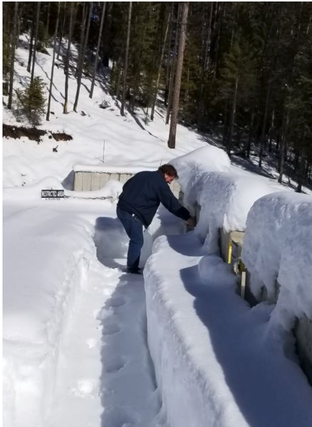
Pressure testing at Flower Creek Dam, winter 2019
