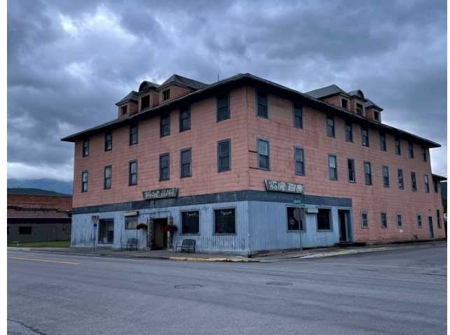
Hotel Libby, an underutilized, historic building
