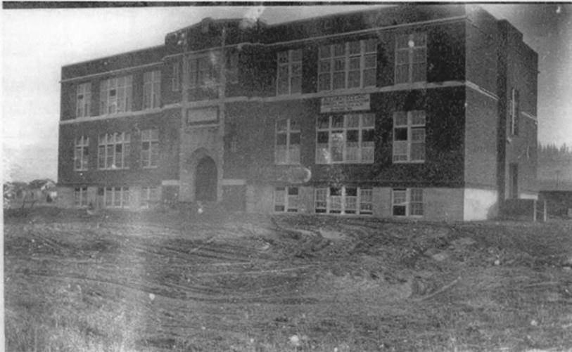
Libby High School under construction in 1916. View to south.
