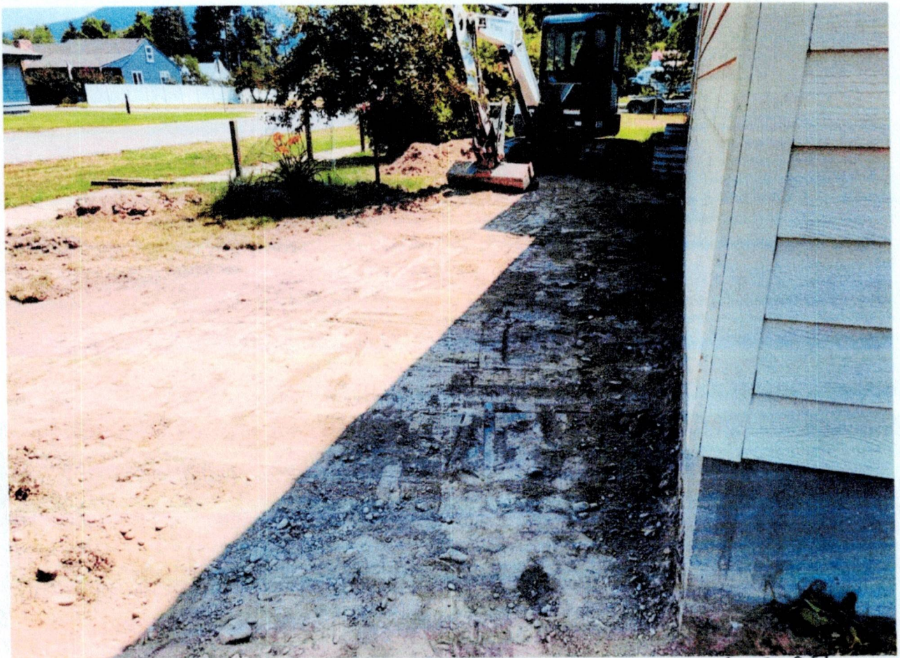
Posts Remain in Ground July 13 2023
