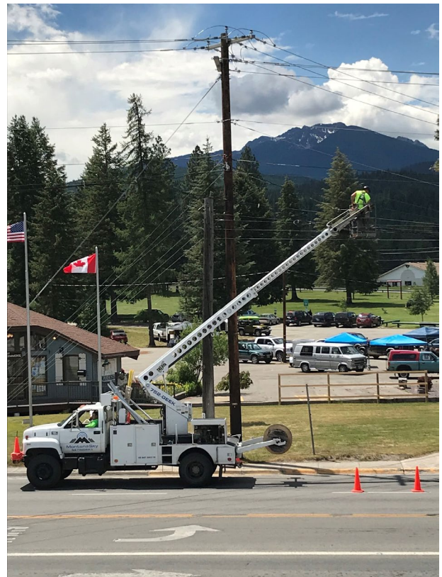
Montana Sky servicing overhead utilities; photo courtesy Amber Pacheco-Holm, Montana Sky
