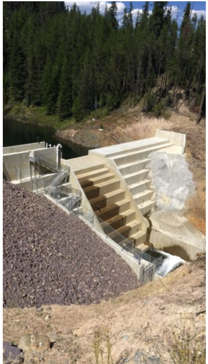
The new Flower Creek Dam near completion
